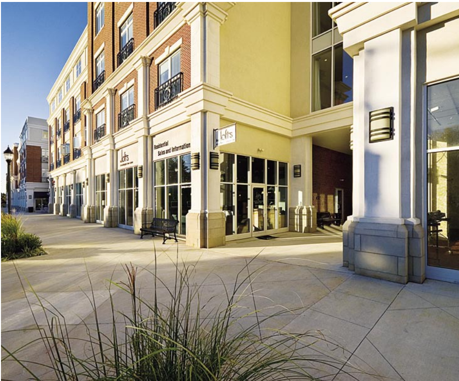
Sharbell's Washington Town Center in Robbinsville, NJ, is a special mixed-use development featuring a great combination of retail and residential components.
